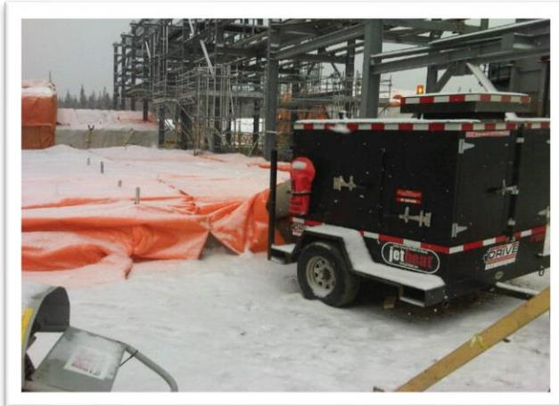
*A CH15HS heater thawing out a large area of ground at a construction site in winter*
